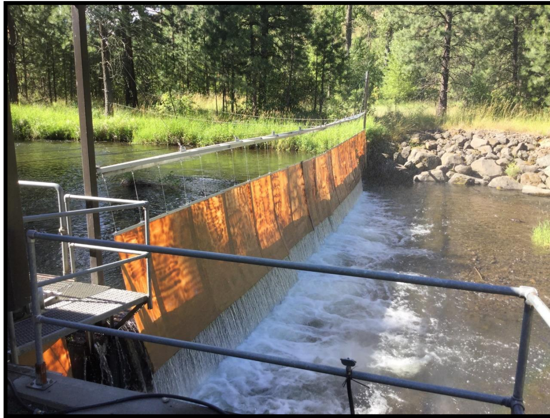
Figure 5: Tucannon River Project Area 13 pre-project conditions in 2018. The upper left image is the Tucannon Fish Hatchery weir and fish trap located at the upper most end of the project area. The project reach is described as a combination of plain bed riffle and rapids (lower left and right images) caused and maintained by river levees and riprap. The upper right image shows one of the river levees being removed in 2021 as part of the restoration project design for this reach.
